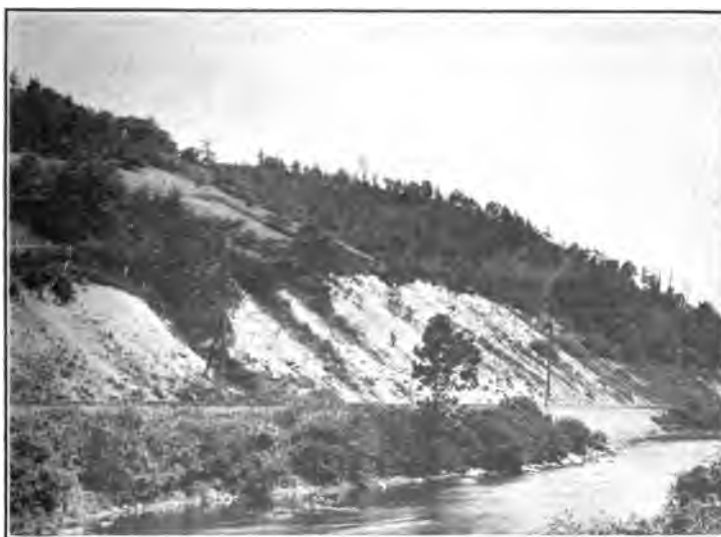
FIG. 38.—Cutting through fag-end of delta, Emporium Junction, Cameron Co.
